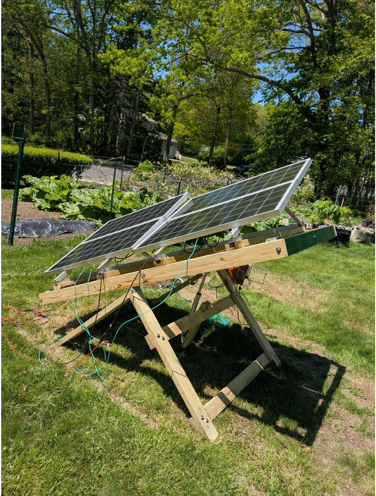
Figure 2-13. Base with Panels Mounted Outside, Front View.
