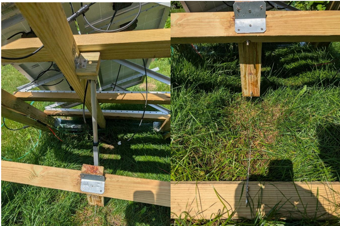
Figure 4.1-4. Additional Support Corner Joint is Bent to the Correct Angle. A wire connected with 2 eyebolts prevents the bottom of the actuator mount from being pulled up.
